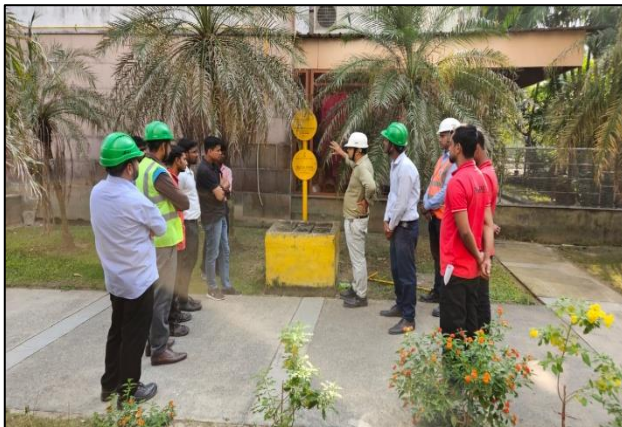
Briefing the location of MDPE Pipeline, Valve chamber and dial before digging
